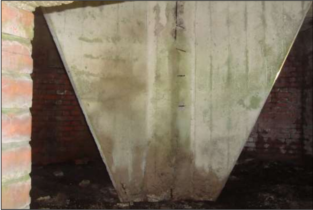
Plate 52: The internal 'Y' shaped anti-ricochet wall
