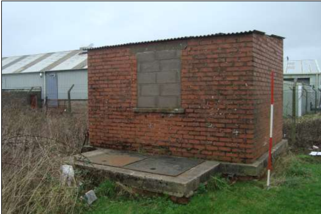
Plate 103: Remains of the MT Petrol Installation structure
