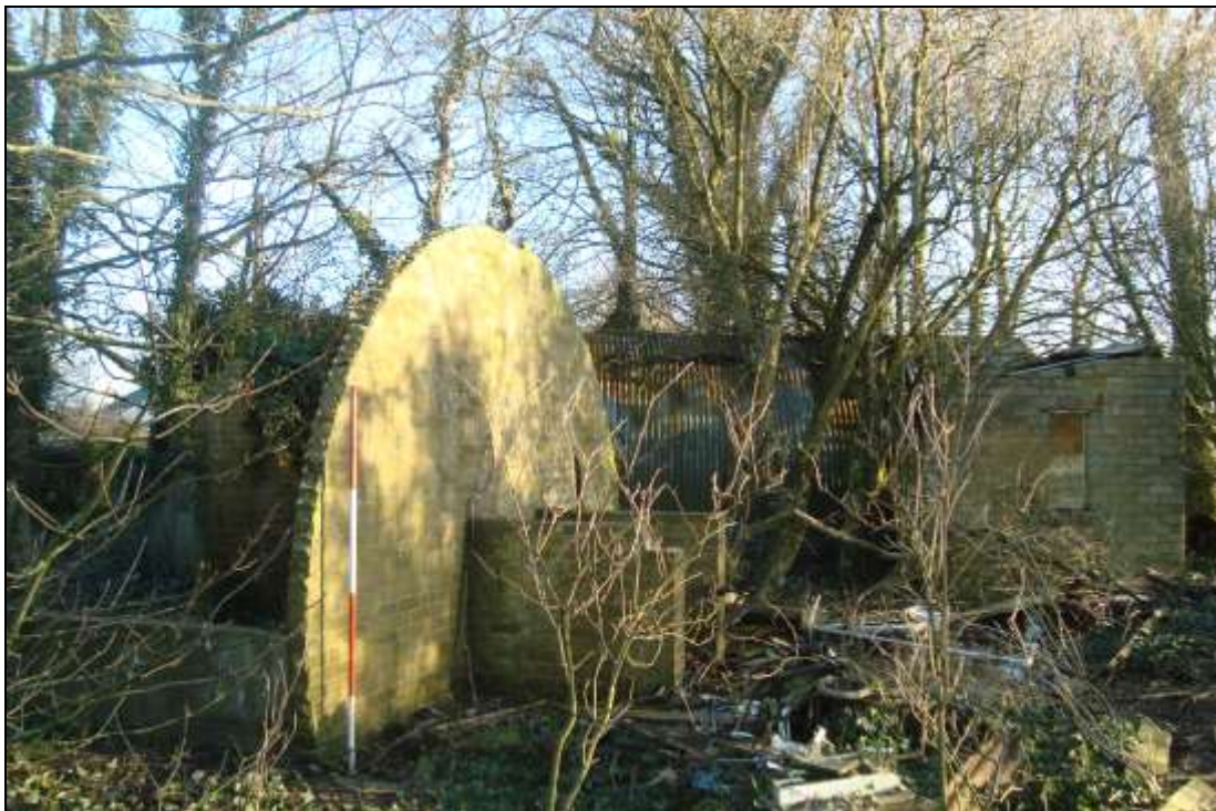
Plate 84: Remains of one of the Turner curved asbestos hutting
