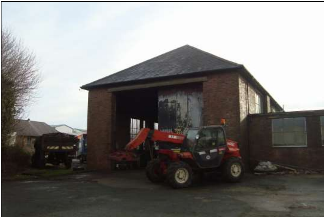
Plate 60: Rear elevation of the Workshop. View to the southeast
