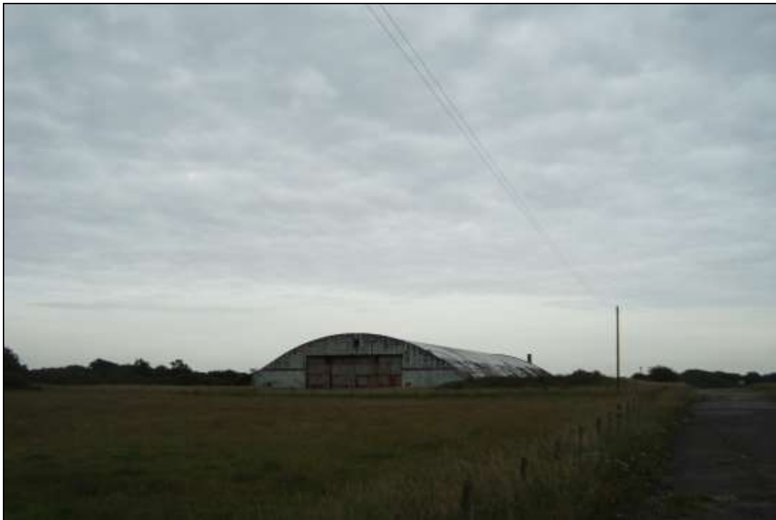
Plate 21: 'L' type hangar 31. View to the south
