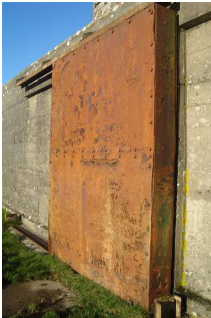
Plate 57: Large cast-iron plates form the sliding door.
