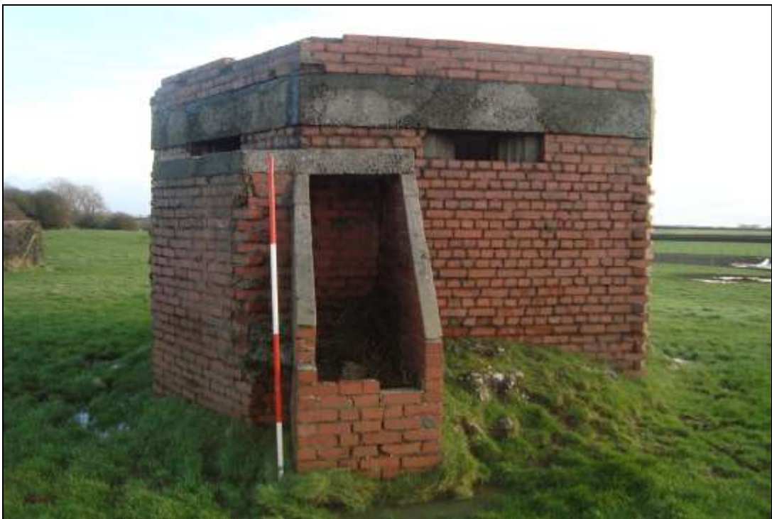
Plate 51: West facing elevation. Note the height of the reinforced entrance.
