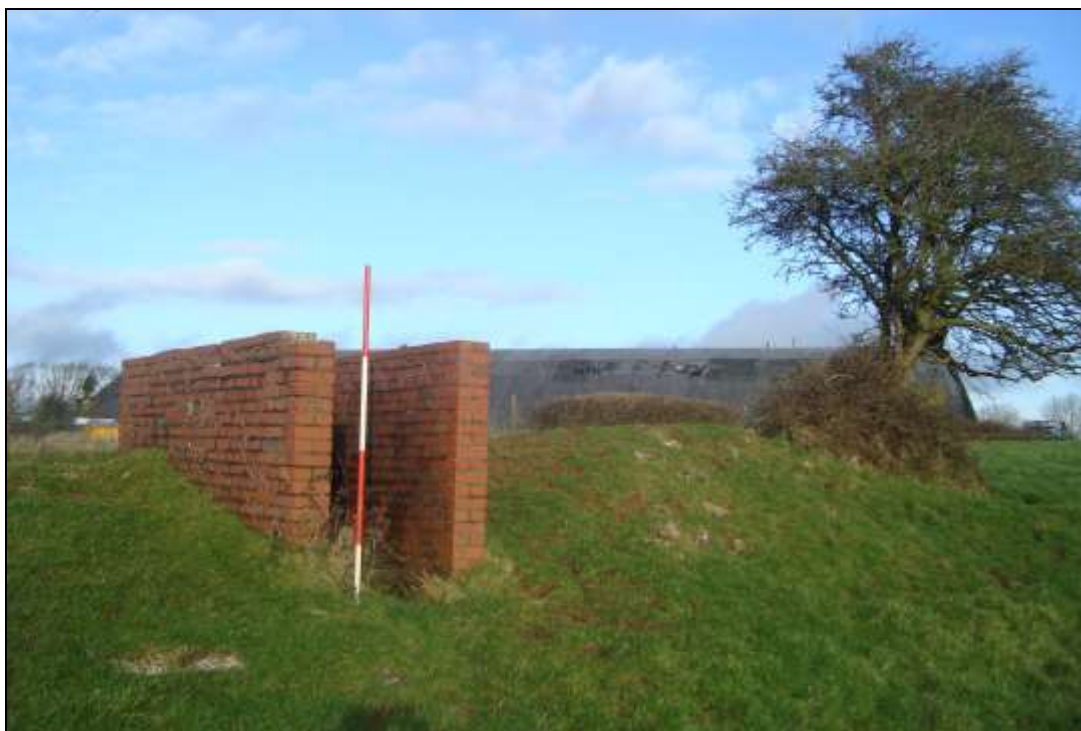
Plate 47: 'Stanton' type air raid shelter. View to the northeast
