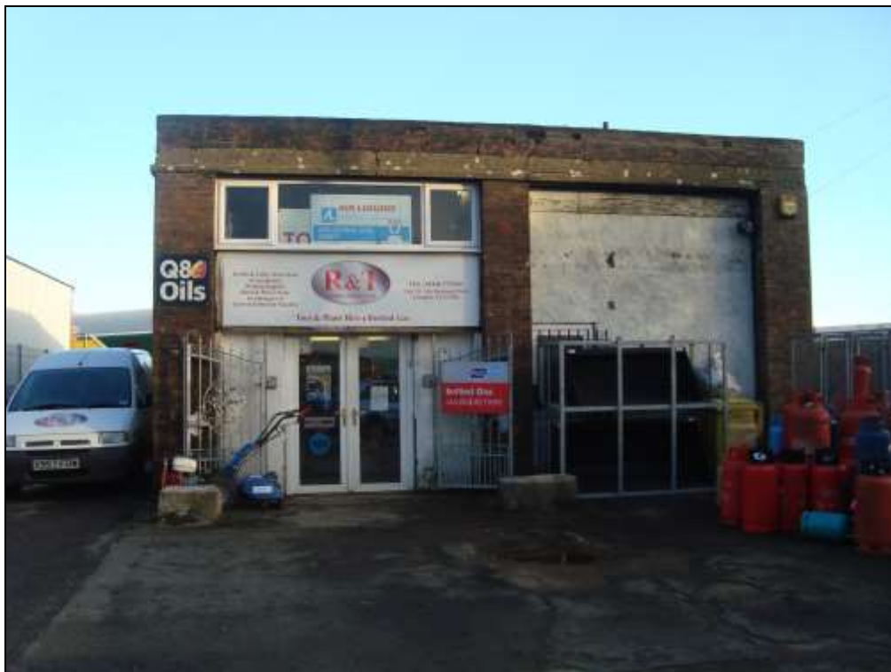
Plate 78: Front elevation of the shed. View to the east
