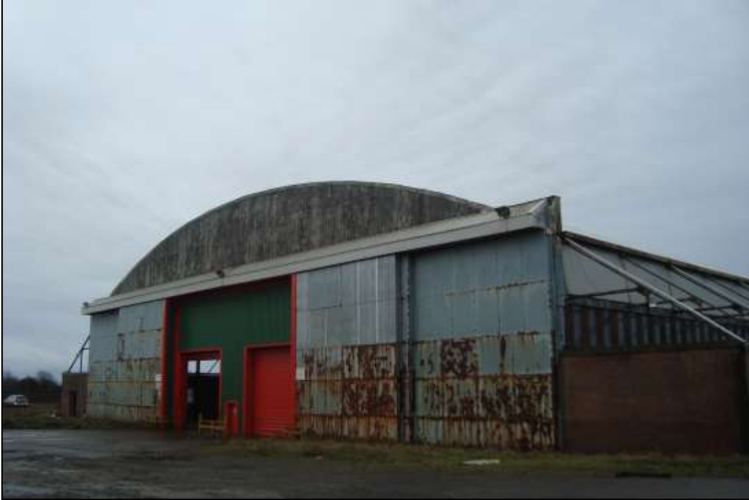
Plate 24: Front elevation of hangar 50. Note the addition of the new door portals
