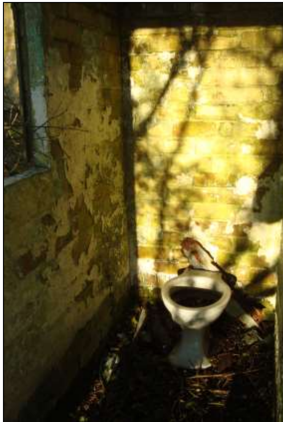
Plate 85: Remains of the latrine block
