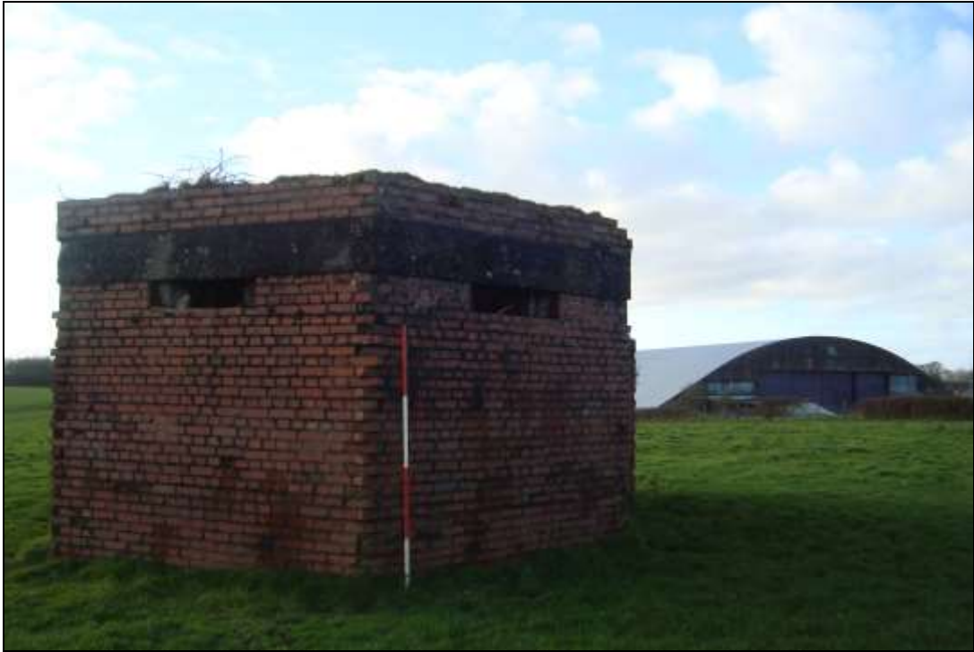
Plate 50: East facing elevation of the pillbox with hangar 62 in the background
