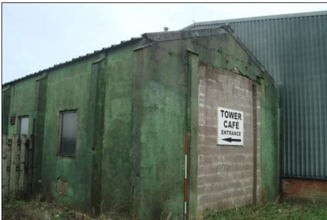
Plate 92: The main entrance bay for the floodlight trailer shed. View to the west
