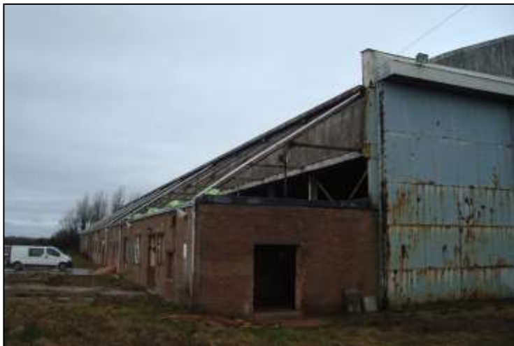
Plate 27: Steel flying buttresses extend out from the roof of the hangar along either flank
