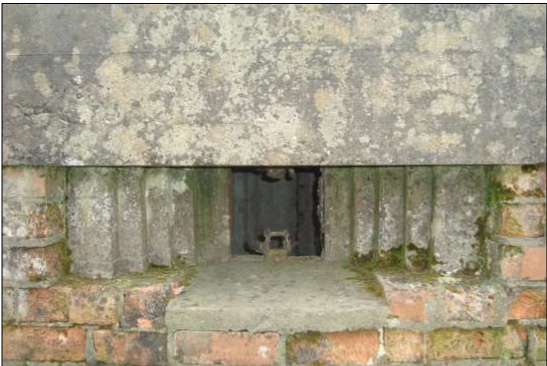
Plate 19: View of the Turnbull mount frame within the northern most loophole
