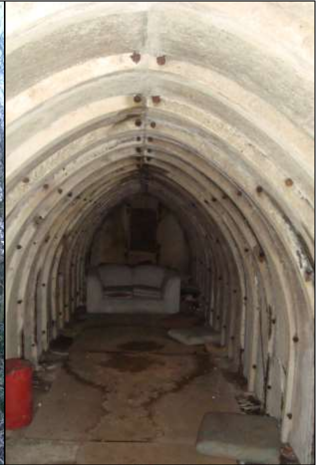
Plate 14: Interior of the shelter. Note the pre-cast rib construction
