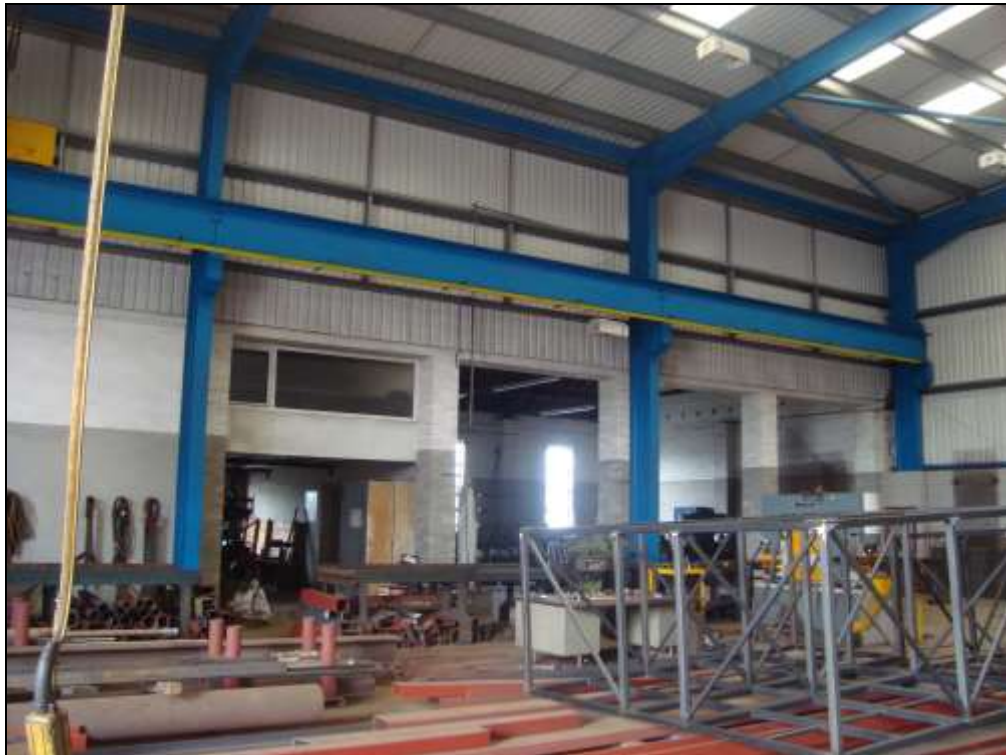
Plate 71: Interior of the building that now covers the MT yard. Note the surviving vehicle bays
