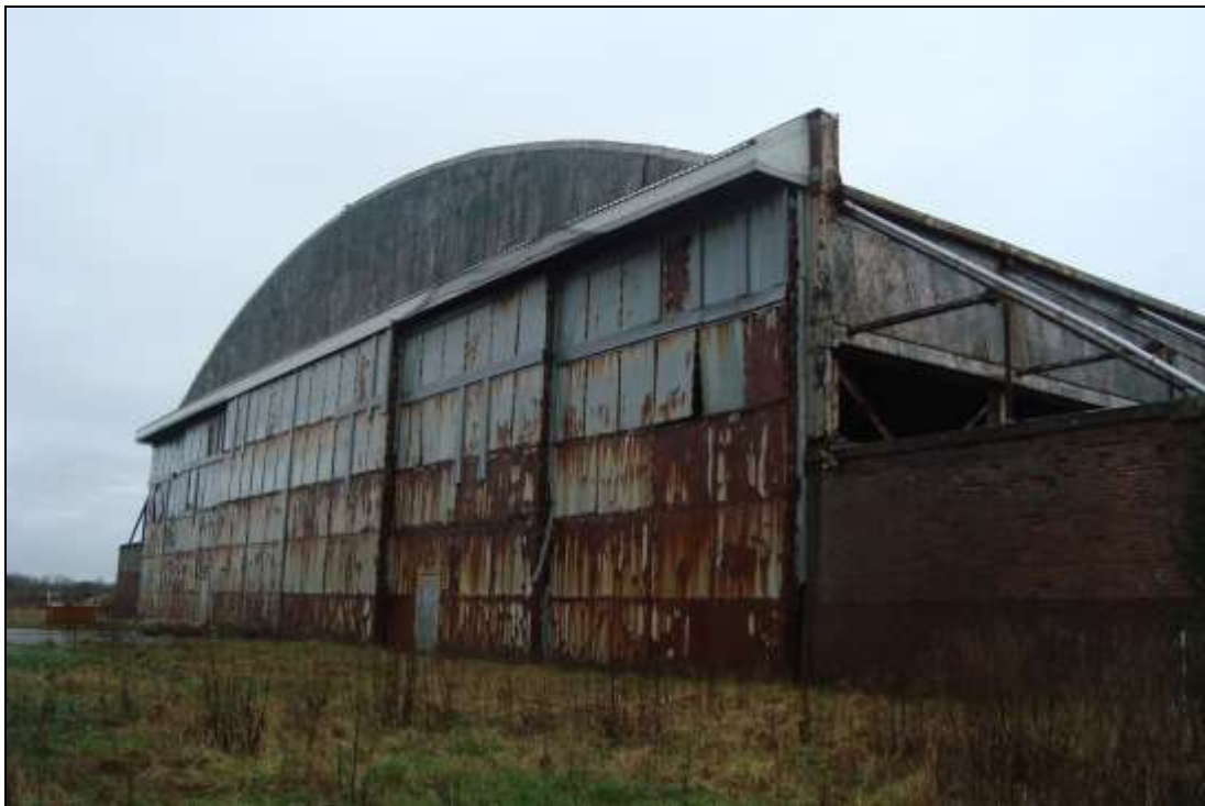
Plate 25: Rear elevation of the hangar
