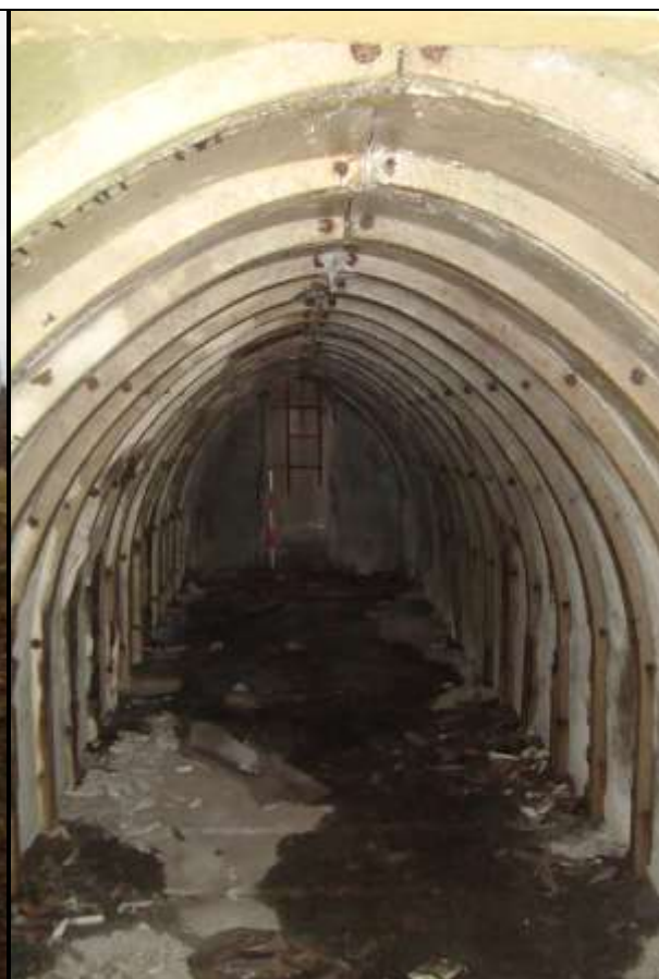
Plate 32: Interior of the shelter. Note the pre-cast rib construction
