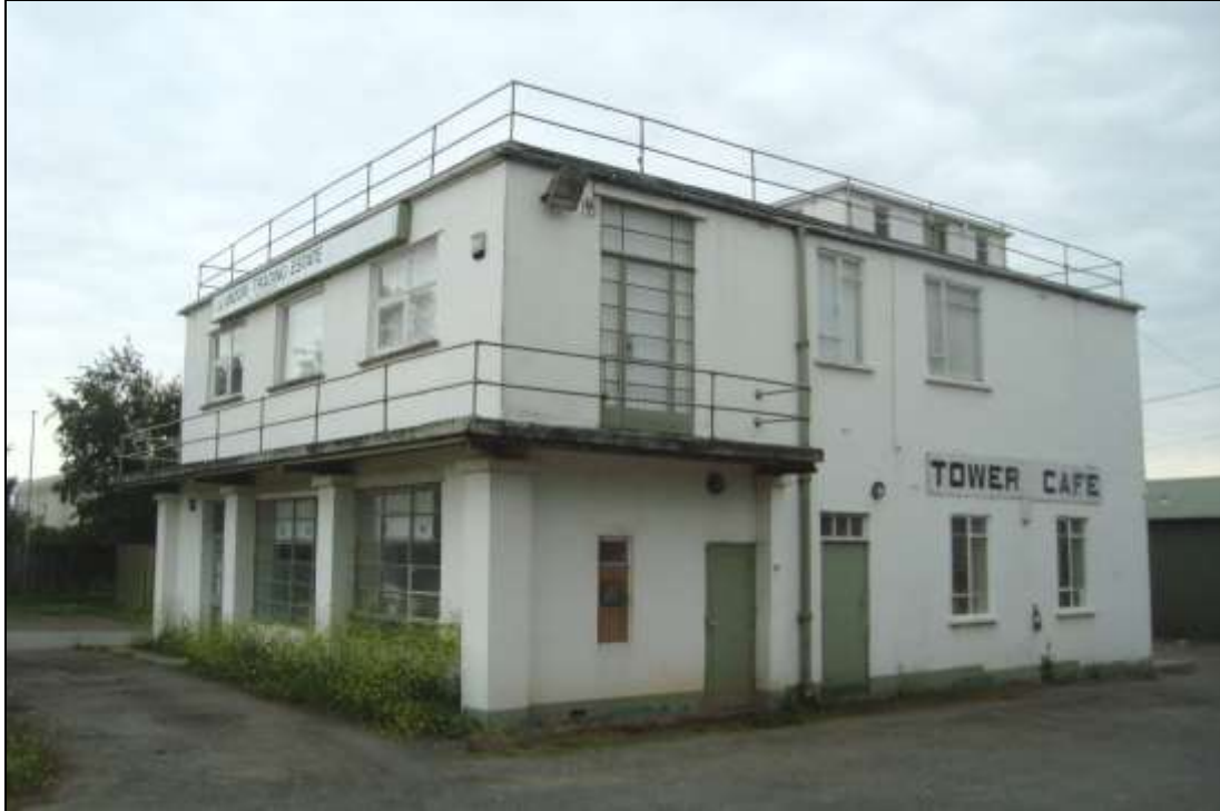
Plate 90: Watch Office at RAF Llandow. View to the southwest
