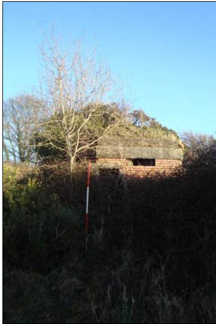
Plate 55: West facing elevation of the pillbox
