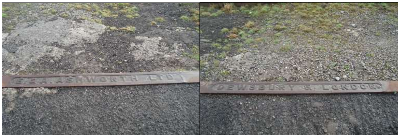
Plate 34: Etched makers name around the cast iron weighing plate frame
