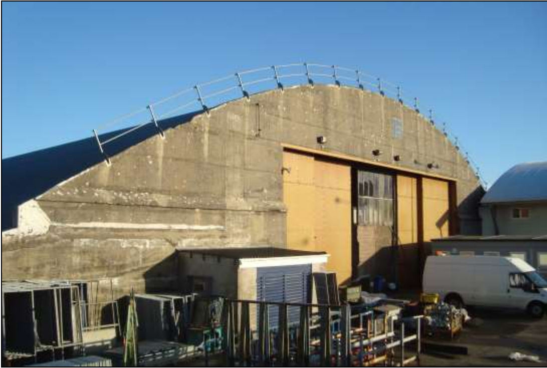
Plate 45: Front elevation of hangar 60. View to the southeast
