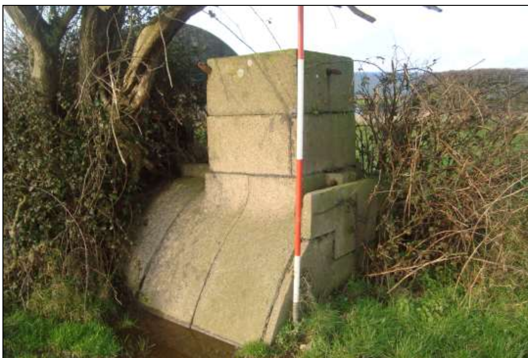
Plate 48: The exposed emergency exit at the eastern end of the shelter
