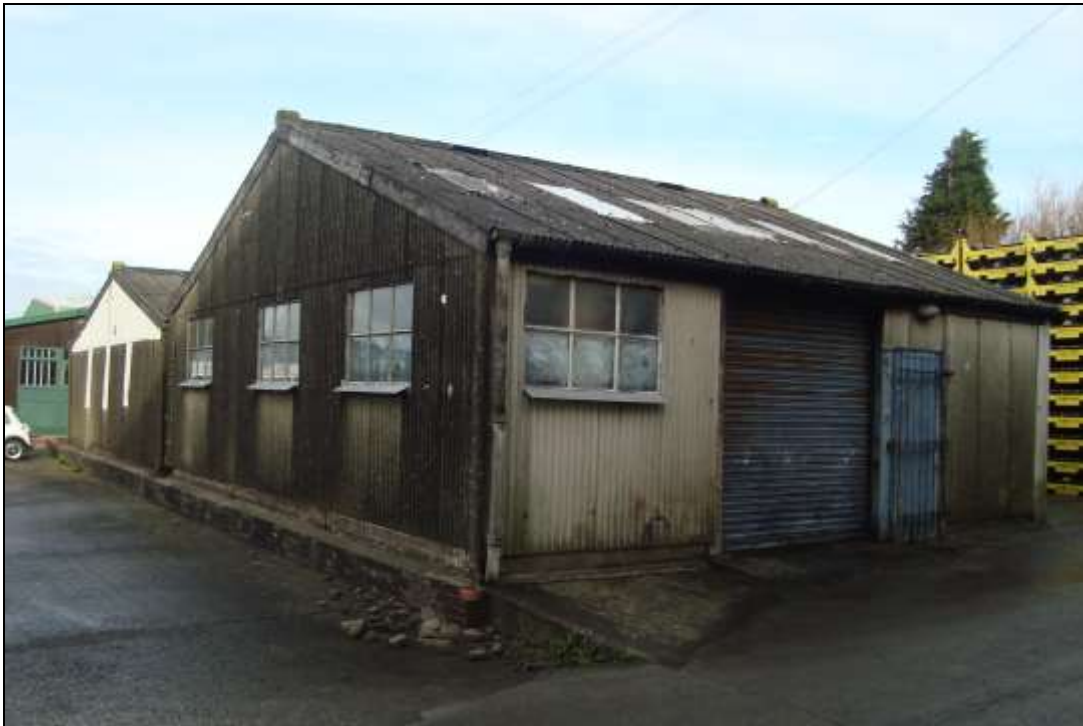
Plate 63: The two prefabricated storage sheds. View to the north
