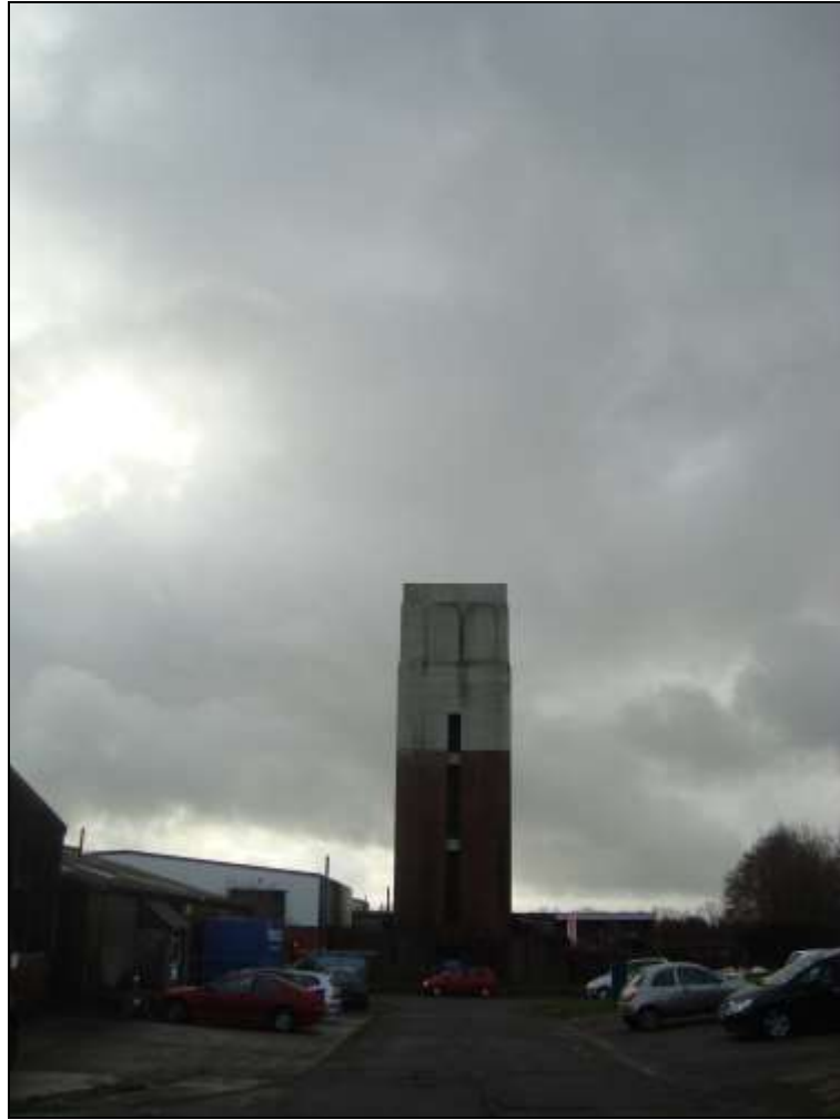
Plate 70: Expansion Period designed Water Tower (north facing elevation)
