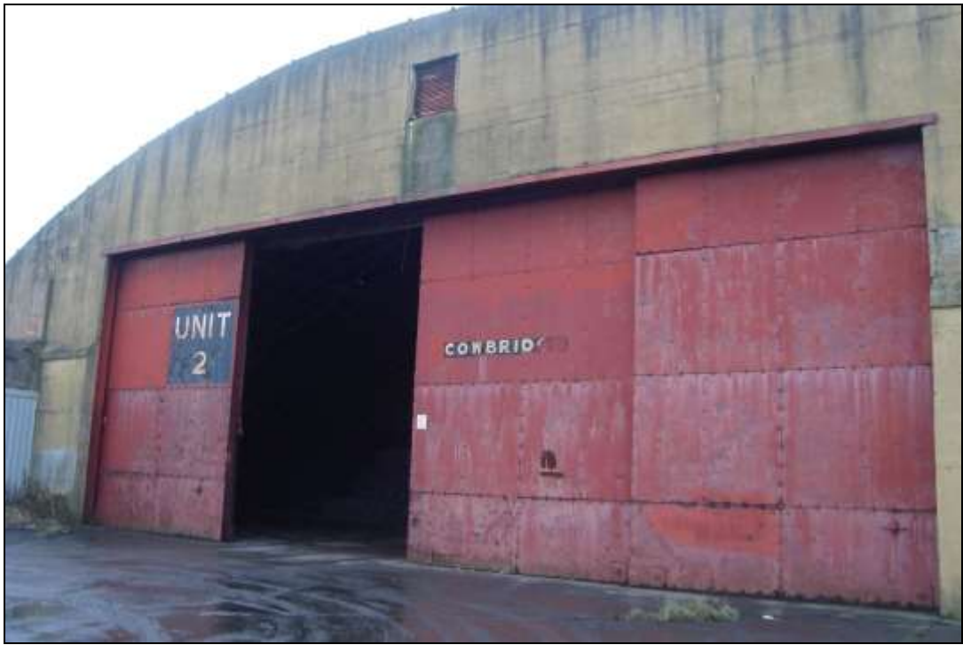
Plate 10: Close-up of the hangar doors
