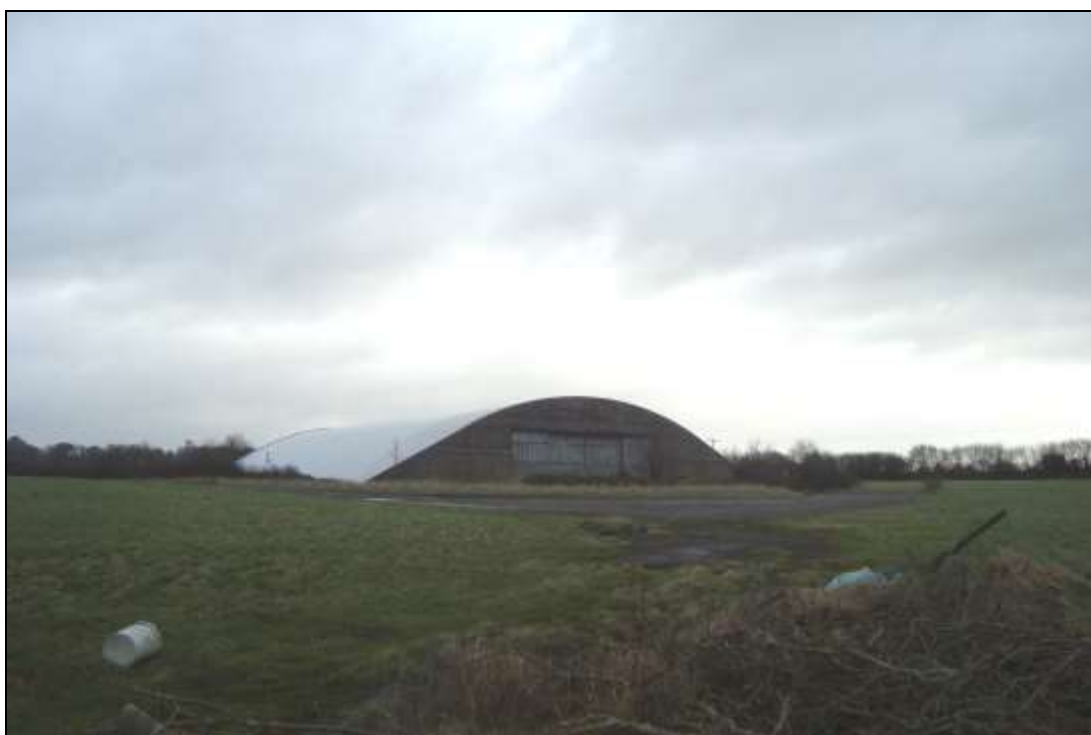
Plate 8: Rear elevation. View to the east
