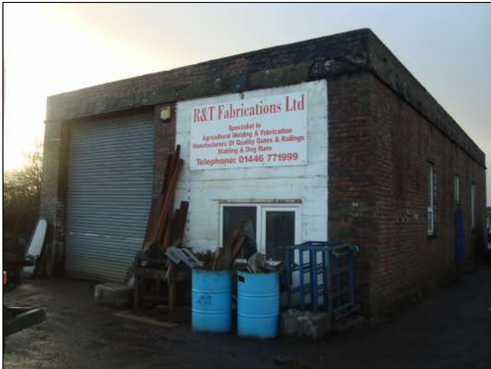
Plate 79: Rear elevation of the shed. View to the west
