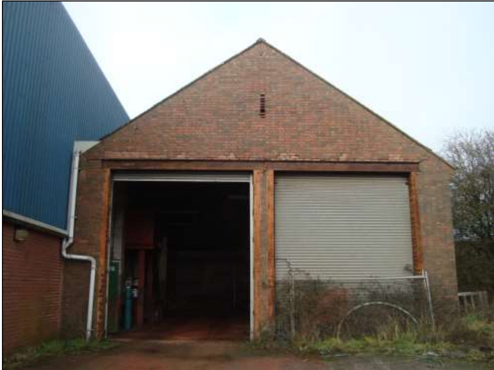
Plate 72: The front elevation of the eastern most MT shed. View to the north.
