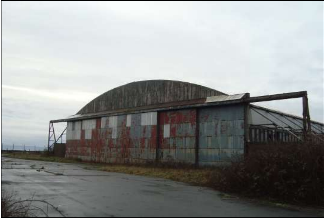
Plate 29: East facing elevation of the hangar with the external outriggers in place
