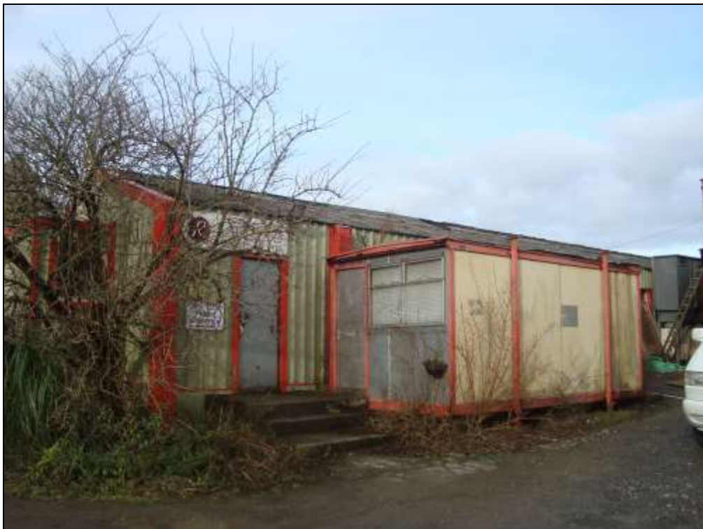
Plate 68: The eastern of the two re-clad Barrack Huts
