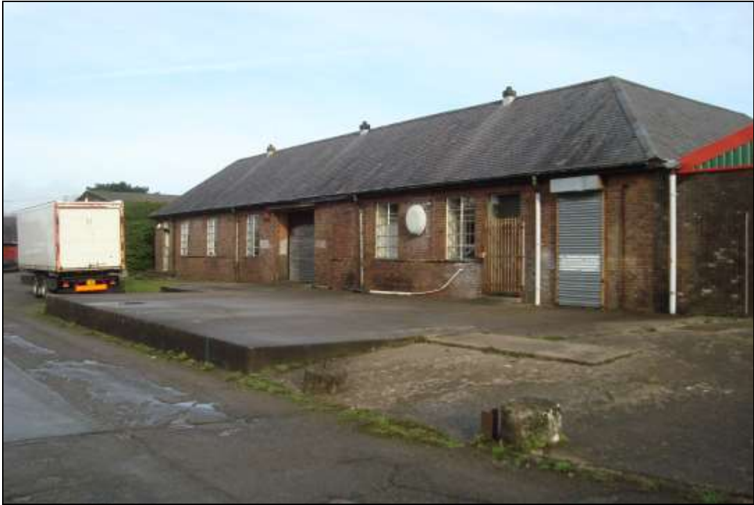
Plate 61: Front elevation of the Canteen Block. View to the north
