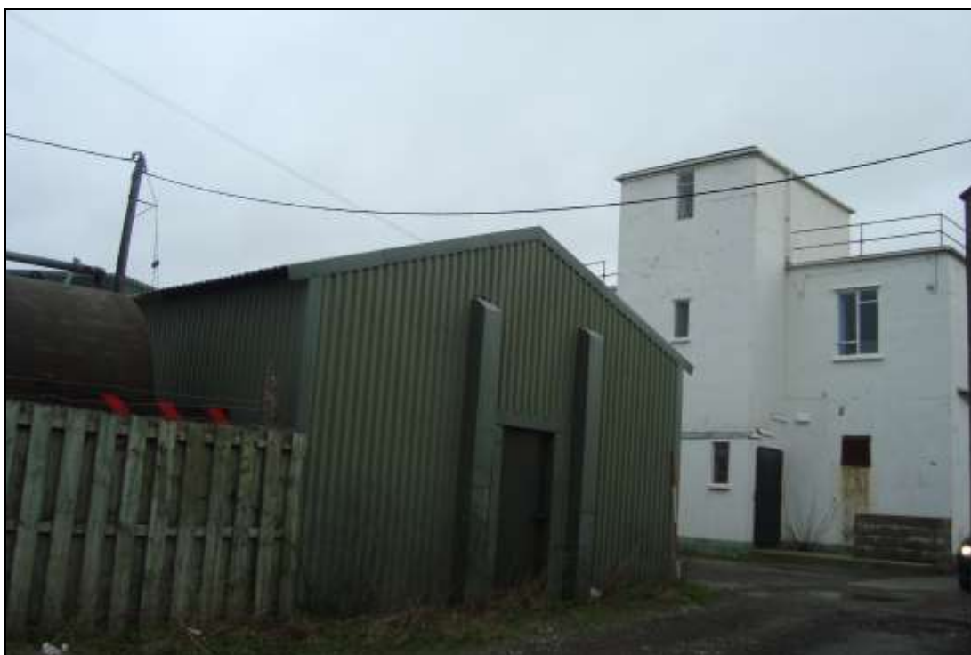
Plate 93: The rear elevation of the building. View to the east.
