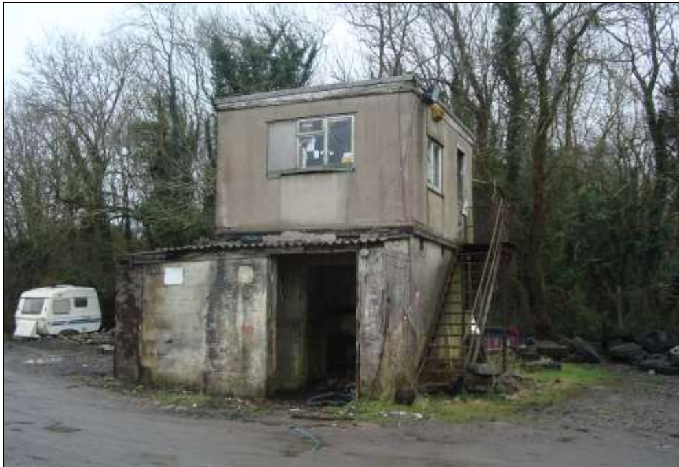
Plate 99: Remain of intake sub-station. Note the later addition to the building.
