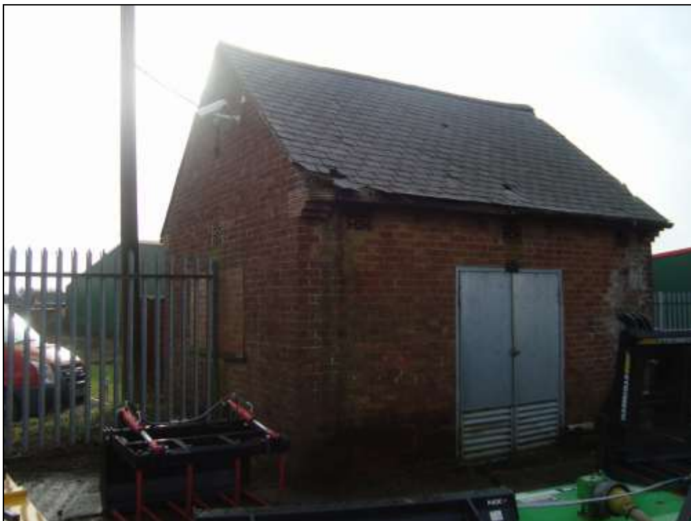
Plate 74: The main compressor building
