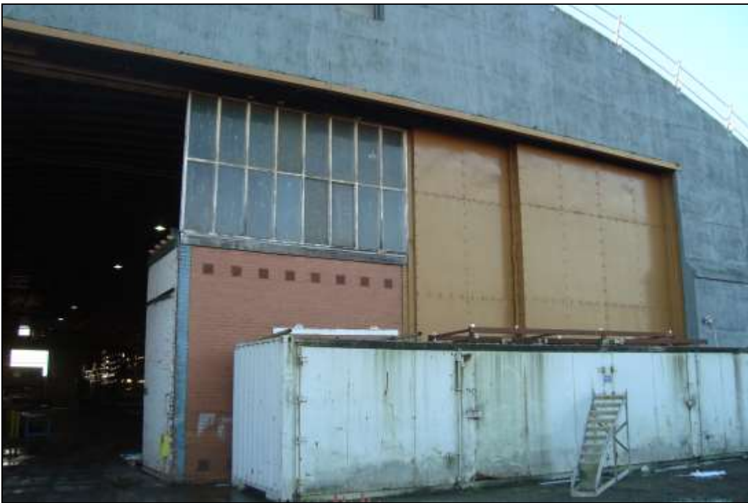
Plate 46: Rear elevation; note the addition of the central brick feature and upper set of windows to the hangar
