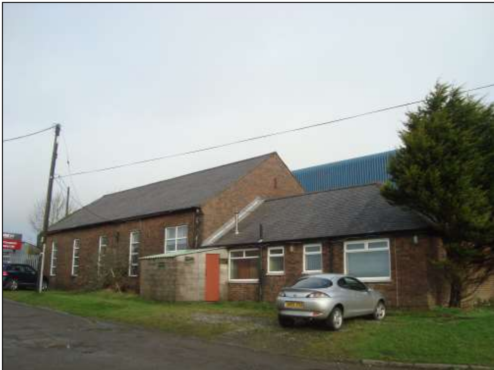
Plate 73: The western MT shed. Note the office building on the right
