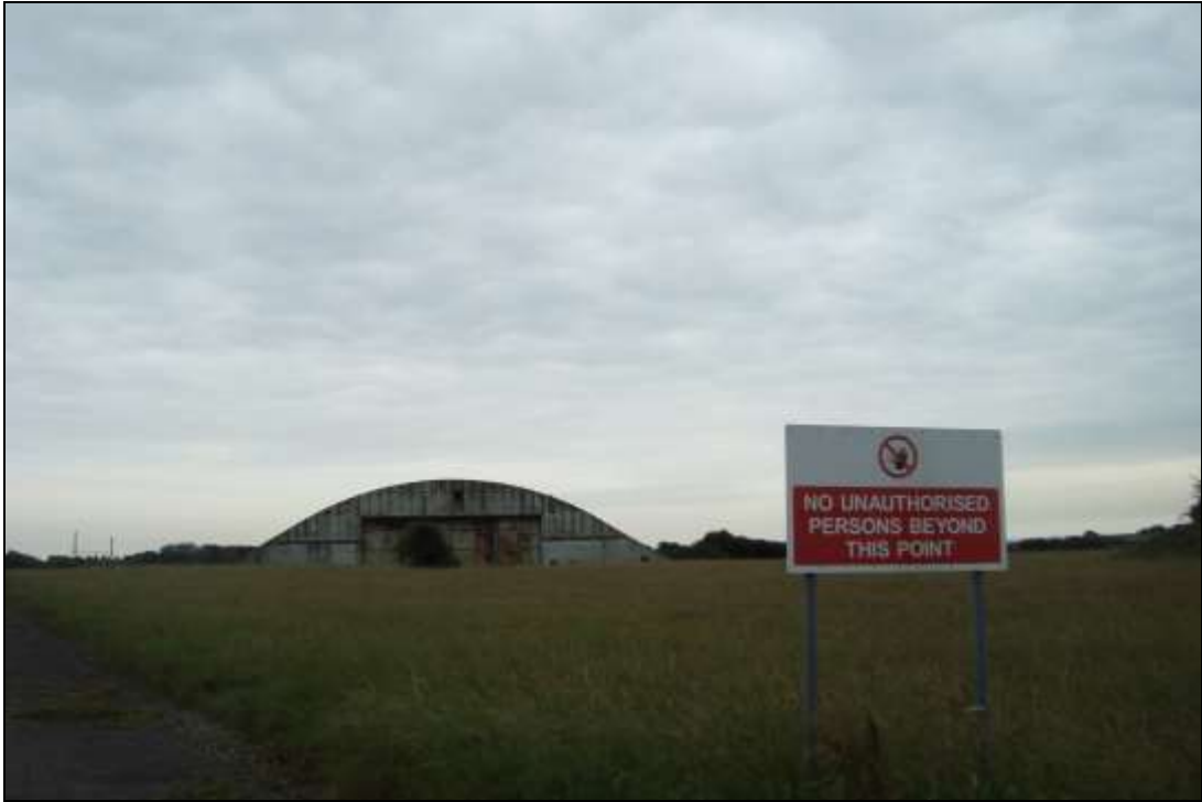
Plate 20: 'L' type hangar 40. View to the south
