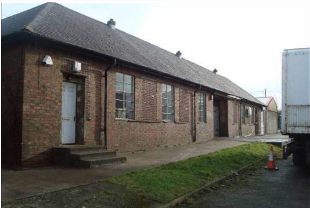
Plate 62: Image showing some of the phasing of the structure. Note the end window has been bricked up before being knocked through and elongated to make room for a new doorway
