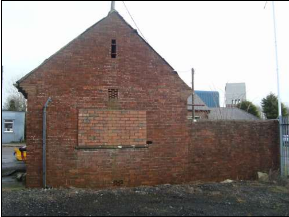
Plate 75: The rear elevation of the compressor house. Note the bricked up window
