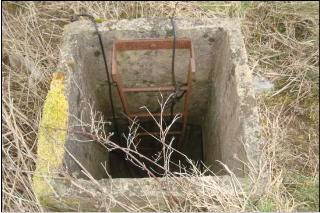
Plate 12: Emergency exit constructed from pre-cast concrete
