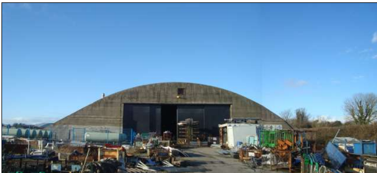
Plate 43: Rear elevation of hangar 61. View to the southeast
