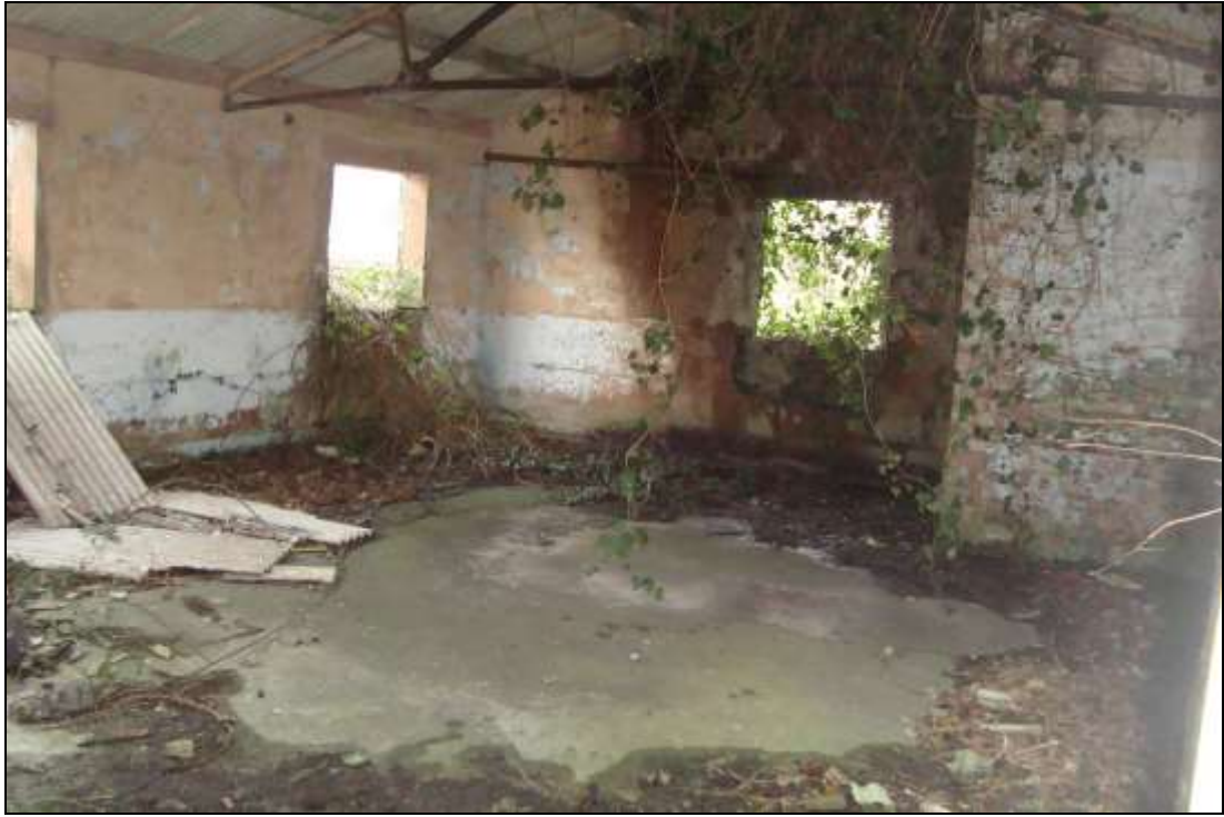
Plate 6: Interior of the canteen. Note the steel 'A' frame roof supports
