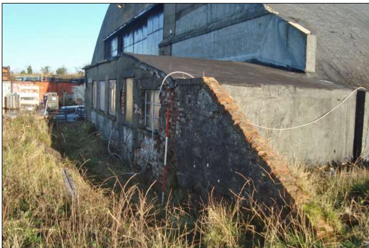
Plate 44: Western office annexe with brick revetment
