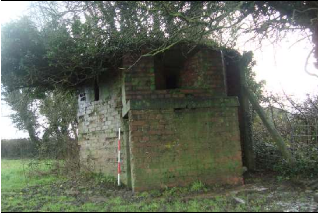
Plate 36: View of the extension, with loophole, above the blast wall (west facing elevation)
