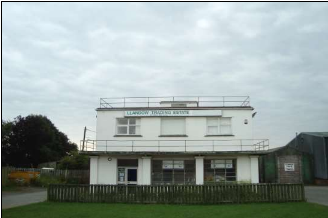
Plate 91; South elevation of the building
