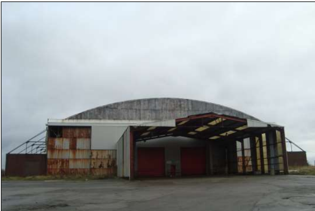
Plate 28: Prefabricated extension to the west facing elevation of hangar 51
