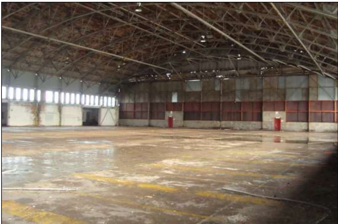
Plate 30: Interior of the hangar. View to the east
