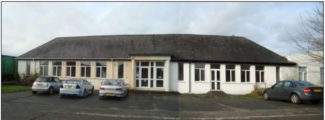
Plate 67: Front elevation of the Station Office. View to the northwest
