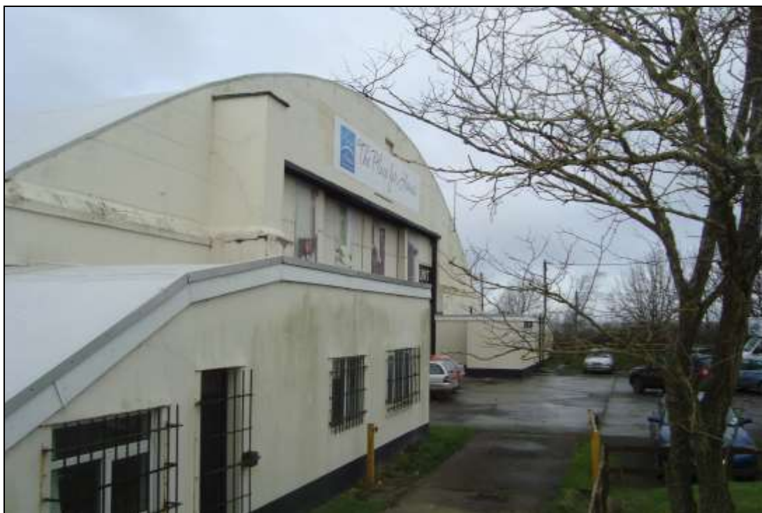
Plate 7: Front elevation of the 'L' type hangar. View to the northwest
