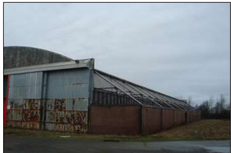
Plate 27: Steel flying buttresses extend out from the roof of the hangar along either flank
