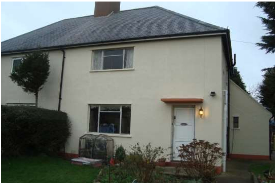
Plate 17: Eastern of the two Married Wardens Quarters (south facing elevation)
