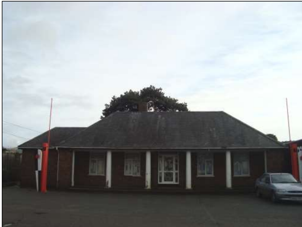
Plate 65: Front elevation of the Wardens Office. View to the east
