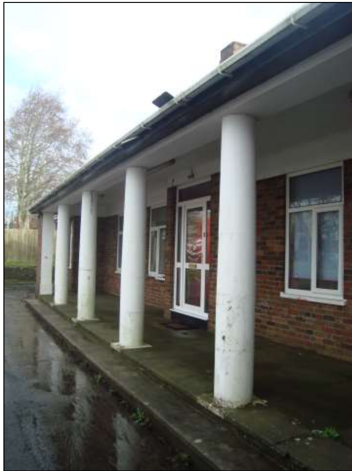
Plate 66: View along the front colonnade. Note the new UPVC windows
