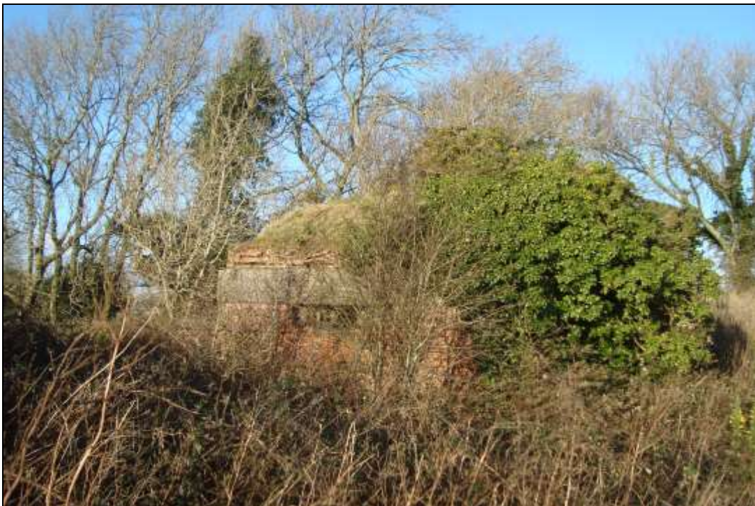
Plate 54: South facing elevation of the pillbox
