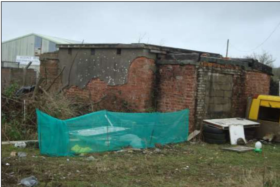
Plate 104: Remains of a transformer sub-station. View to the North
