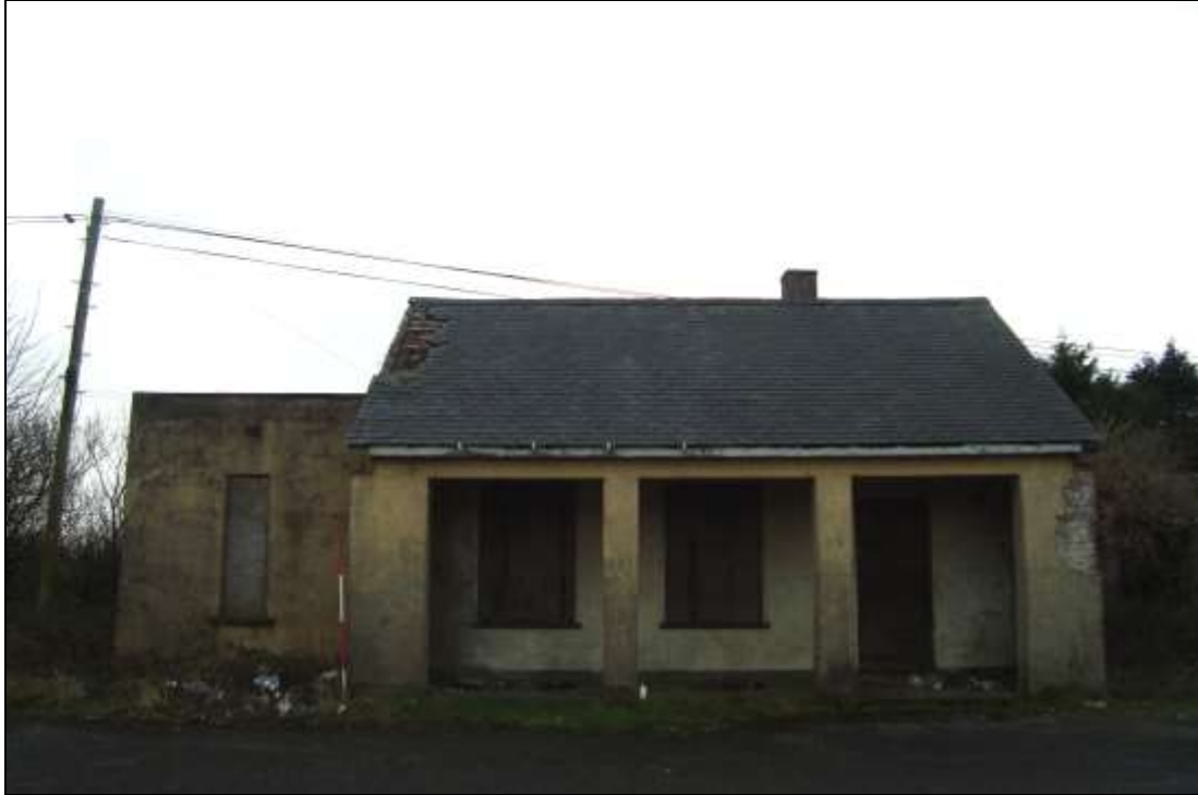
Plate 1: Wardens Office (northeast facing elevation)
