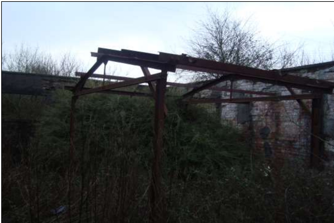
Plate 4: Enclosed area at the rear of the office with the unknown steel framed structure
