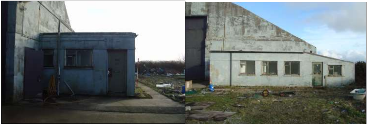
Plate 41: Front and side elevation of the surviving office annex.
