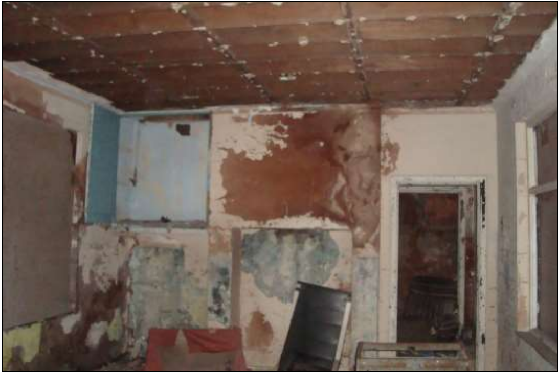
Plate 3: Interior of the building
