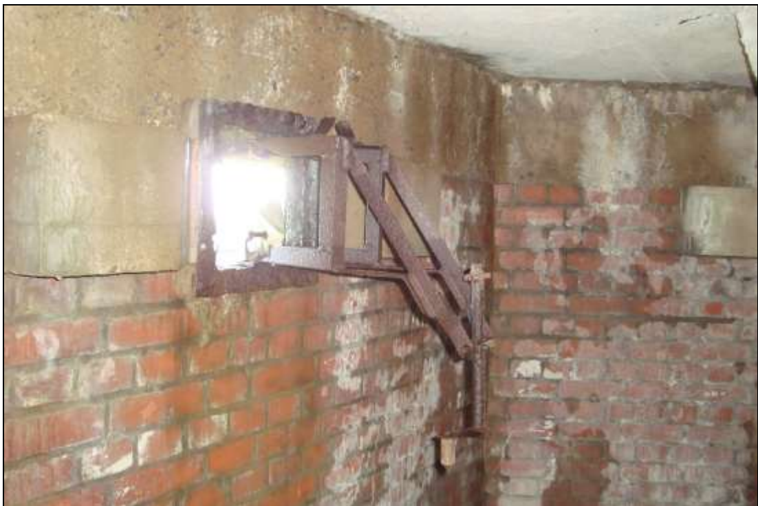
Plate 53: Turnbull mount. Note the wooden handle on the elevation screw still in place.
