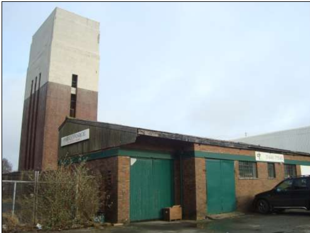
Plate 81: Eastern end of building LD44
