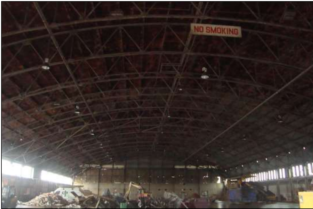
Plate 26: The internal curved steel framed superstructure is still intact
