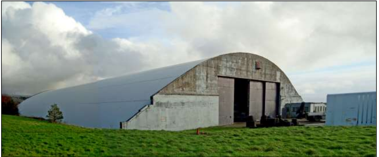
Plate 40: 'L' type hangar 62, main entrance (west facing elevation)
