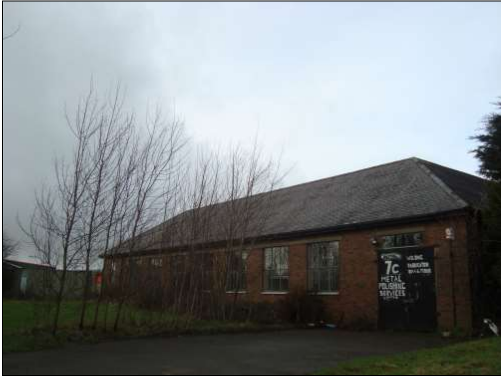
Plate 77: Original windows down the southern annexe (south facing elevation)
